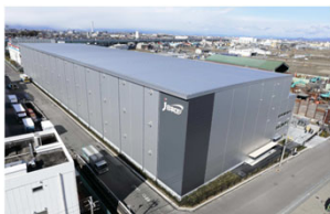
Kiyosu Logistics Center
