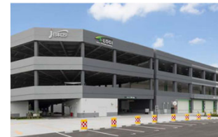
Ichinomiya Logistics Center
