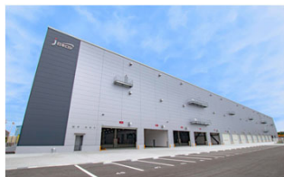
Shiroy Logistics Center
