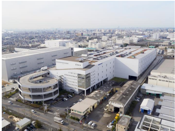
[View of the Facility]
