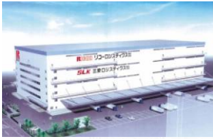
Overall image of logistics center
